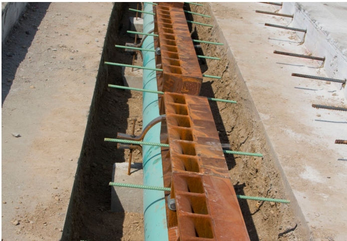
Linear slotted drain vane grate during installation
