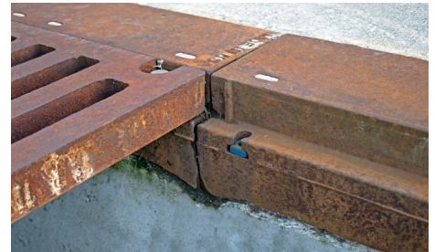
Top flange installed frame
