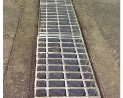
Custom steel replacement trench grate designed to fit existing iron frame.
