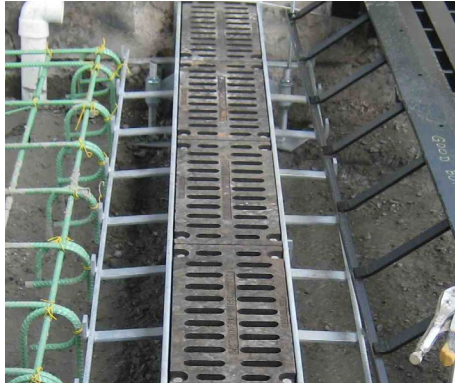
Steel grate frames built to any length of drainage required incorporate cast iron or fabricated steel grates to meet your project needs.
